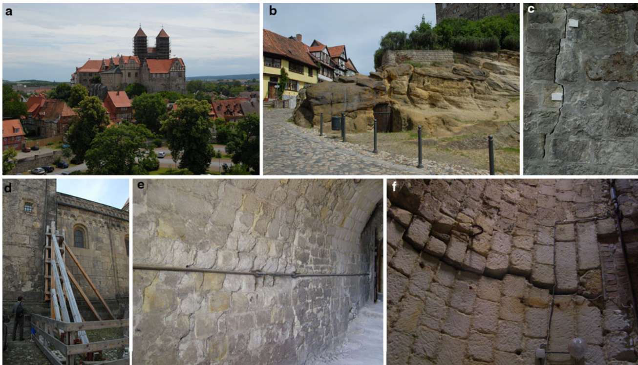
Fig. 1 a View towards the Renaissance-style castle ( left ) and the Romanic collegiate church of St. Servatius located on the top of the castle hill (Schlossberg) in the old part of Quedlinburg. b Slightly cemented early Cretaceous quartz sandstones of the castle hill, which are protected from erosion by a thin conglomerate layer. It contains
