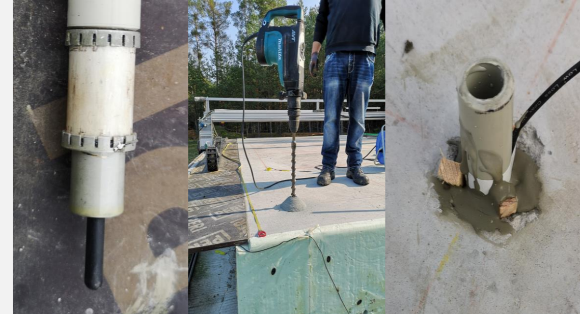
Fig. 1: Embedding of US-transducers and temperature sensors in a large concrete model
