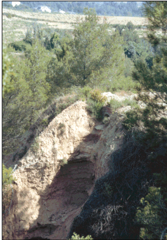
Figure 4.17. Outlet of a drainage channel in a vineyard parcel that has produced a retreat of the gully wall by direct impact of water flow and undercutting of the wall.
