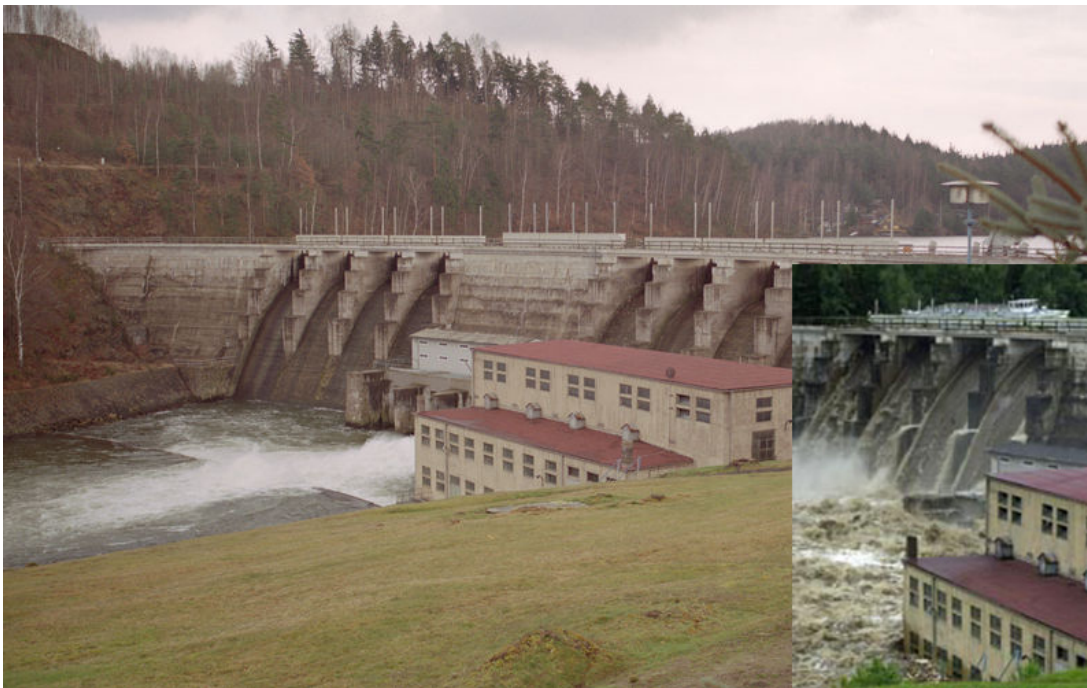
figure 42: Kriebstein dam during the 2002 flood event ( www.wikimedia.de/ www.doebelnerleben.de )
