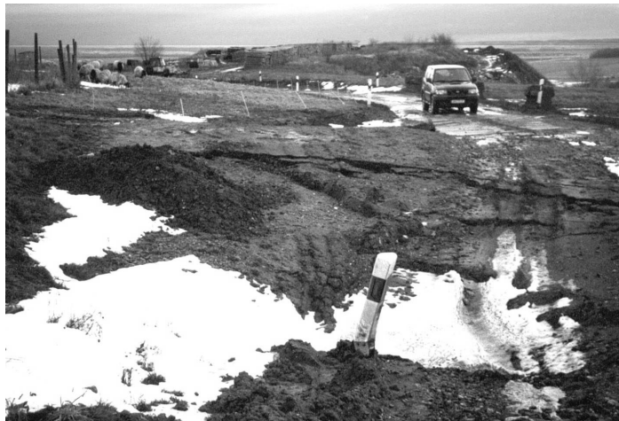
Figure 5.12: A recent ground fall at the salt-waste dump Menteroda
