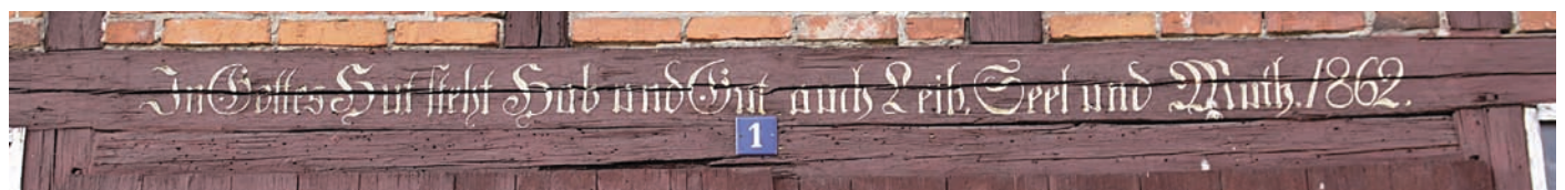
Spruch am Bauernhaus, Güstrower Str. 1 Inscription on farm house, Güstrow Street 1
