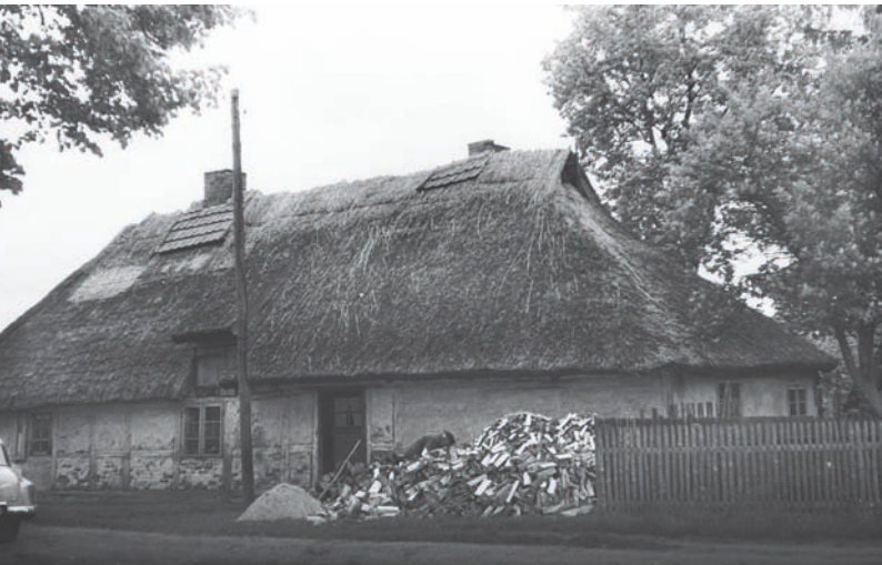
Reet gedecktes Bauernhaus von 1818, Zustand 1968 Thatched farm house from 1818, as of 1968
