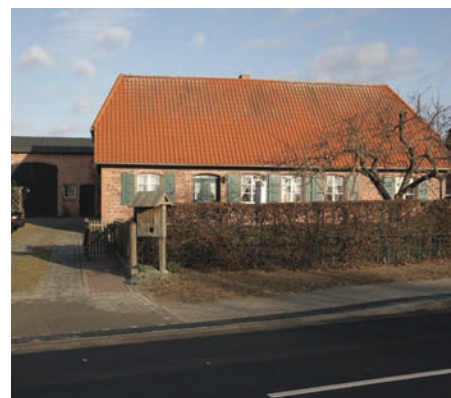
Ehemalige Büdneri an der B 192 Former smallholding (Büdneri) along Federal Road 192
