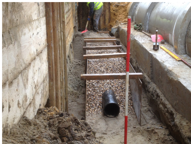
FIGURE 9 Drainage pipe being installed next to a reconstructed sewer pipe (Emschergenossenschaft)
