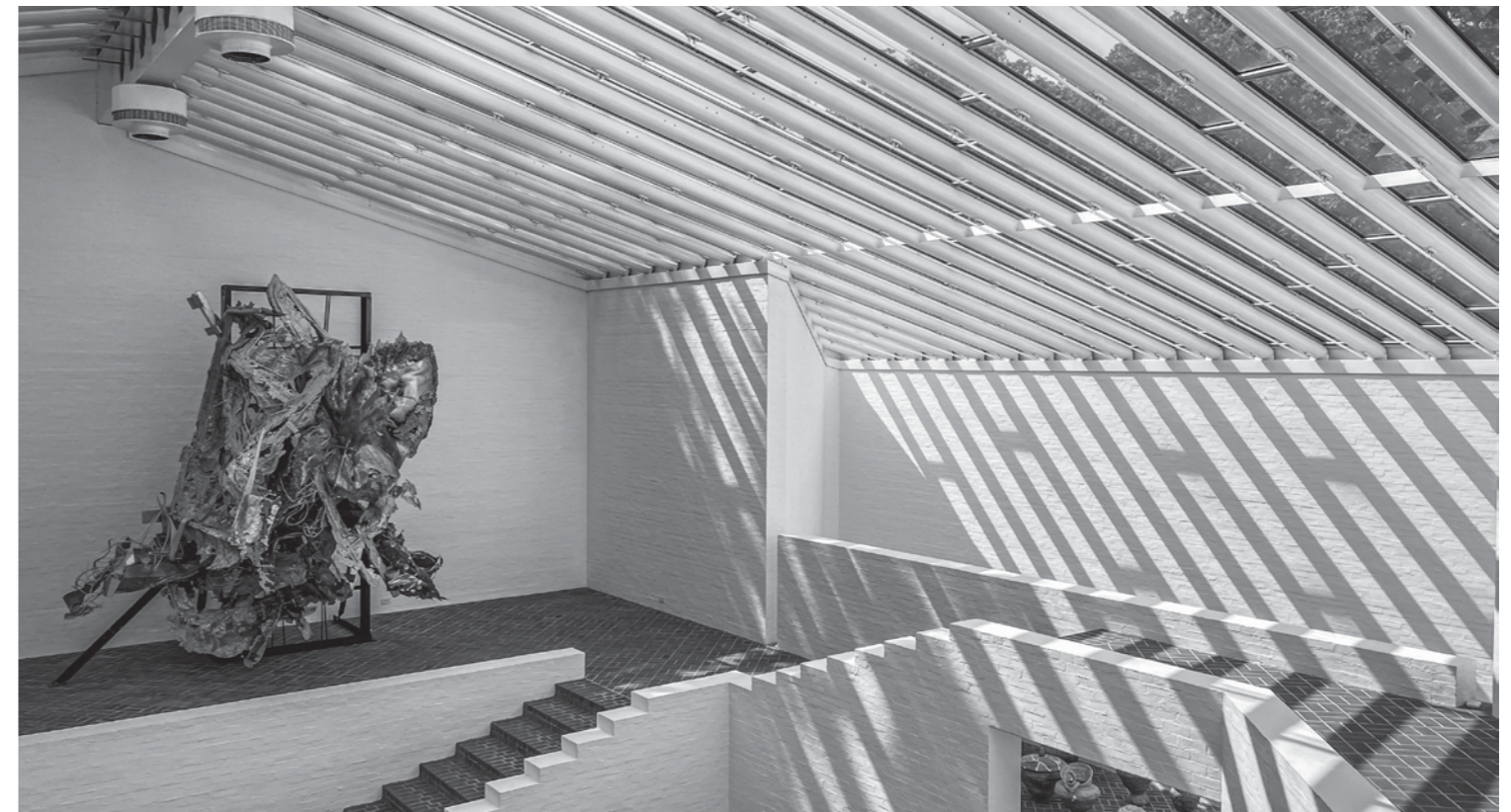
Figure 2.5. The shading structures for glass windows on the surface of the building wall (Source: unsplash.com)
