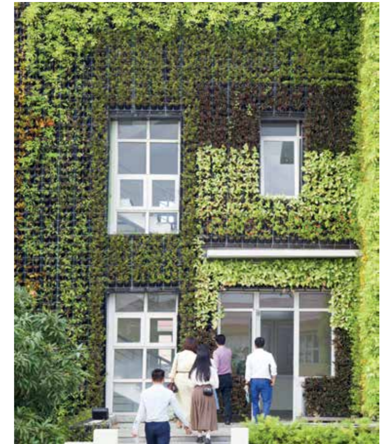
Figure 9.1b. Roof and façade greening is chosen because of low heat absorption compared to other materials like concrete or galvanized steel (Source: Picture left: Michael Waibel, 2023; picture right: © GIZ/Luong Thanh Trung, 2023)
