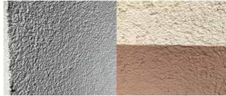
Figure 5.5. Example of two kinds of plaster walls (Source: Andreas Zegowitz)
