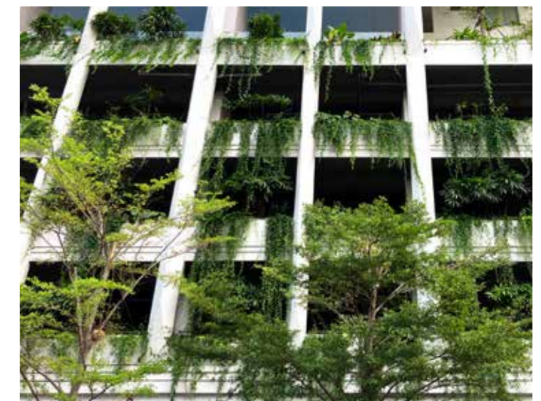
Figure 1.8b. Reducing heat by greening the façade (Source: Michael Waibel, 2023)
