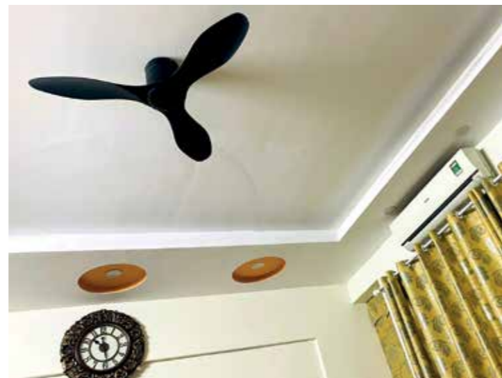
Figure 8.6: Energy saving by using both the ceiling fan and the air-conditioner (Source: Nguyen Huong Lan)
