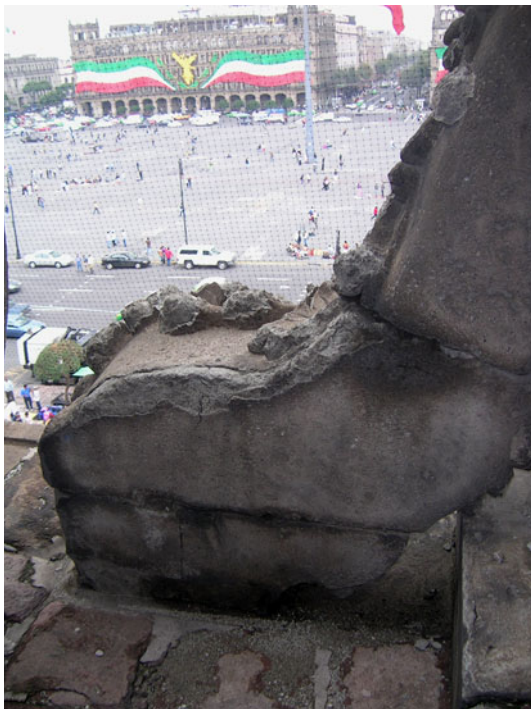
Fig. 4 Crust formation, scaling and rounding of a sculpture at the Metropolitan Cathedral
