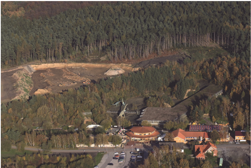
Fig. 6 Overview of the new quarry (upper left, with overburden dumps) and the old one (lower right), rebuilt into the DFM, with the elongated main sauropod track hall. Helicopter photograph, 2005, NLMH.
