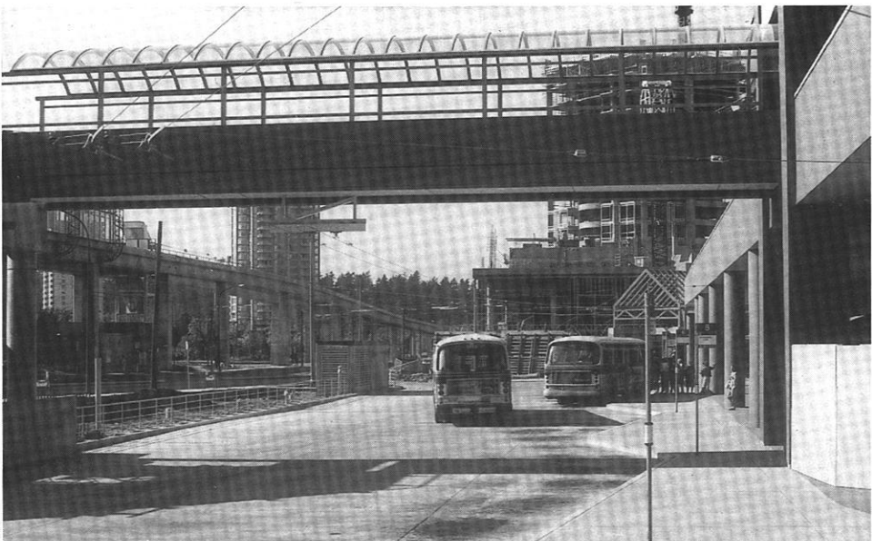
Photo 11: Burnaby's Metrotown station serves as a regional transport node served by numerous bus feeder lines. Aug. 1988
