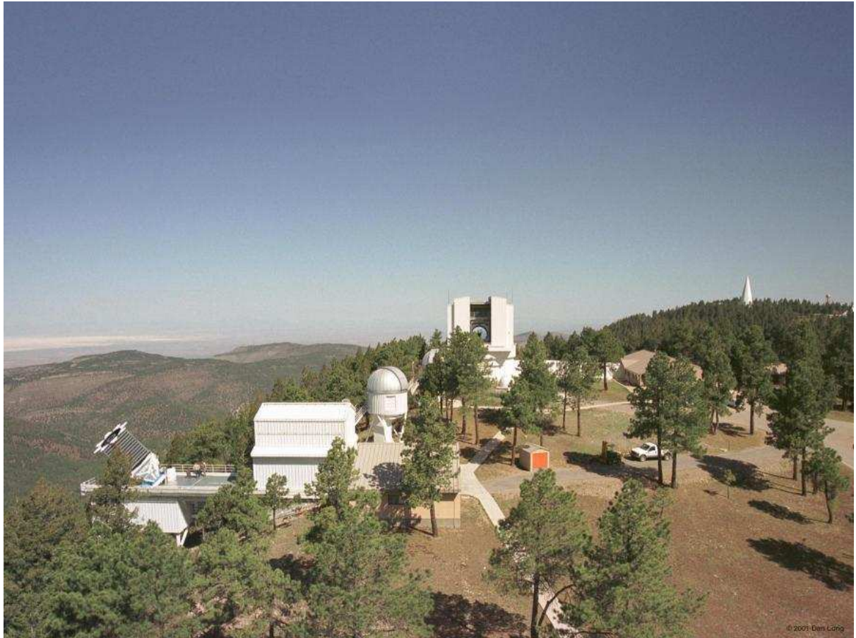
Figure 2.1: The image shows a view of the SDSS telescope site, the Apache Point Observatory, New Mexico / USA (from www.sdss.org ). On the left one can see the 2.5 m SDSS telescope with its removable hut. The light path of the telescope is covered by a wind and light baffle. Near the hut in the foreground, the dome of the photometric telescope is imaged. In the background, the 3.5 m telescope of the Astrophysical Research Consortium can be seen.
