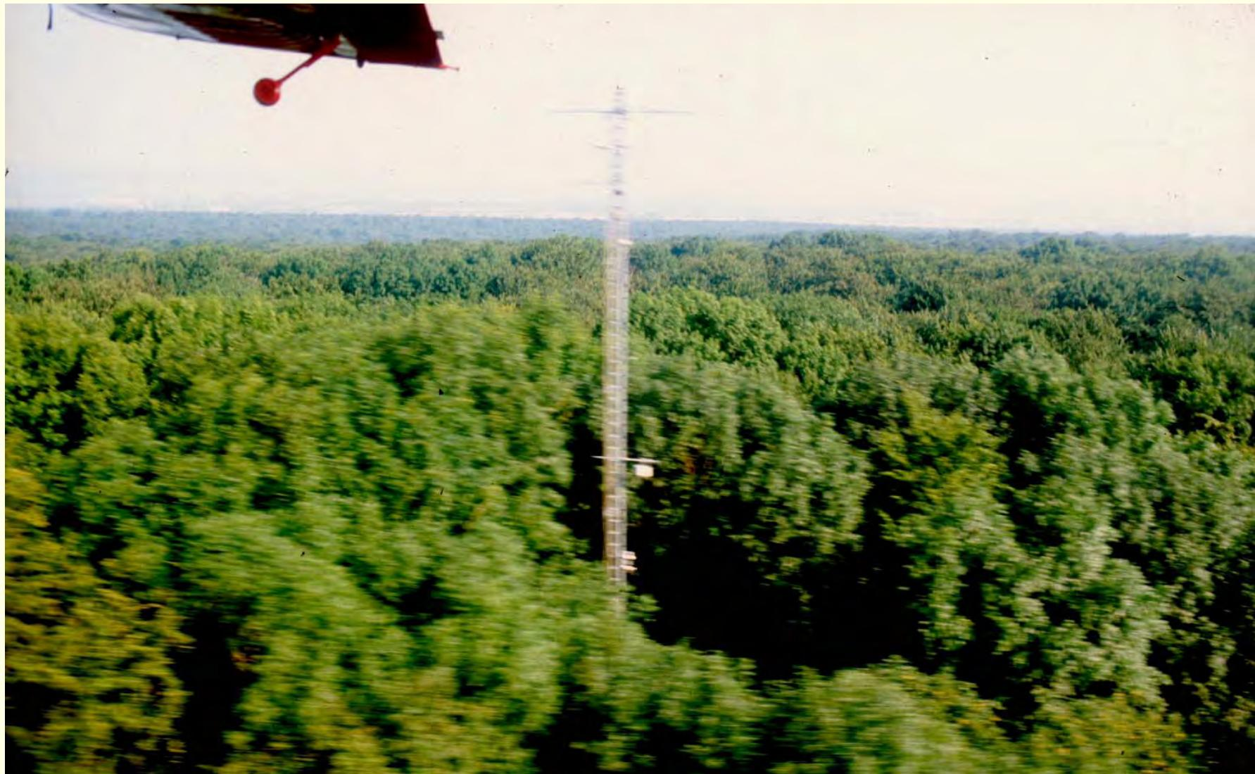
**Figure 9** Hainich Tower (height 42 m, treetops around 35 m). 'Lowest level' sampling altitude approximately 5 - 7 m above the canopy.
