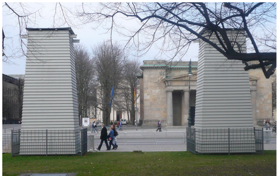
Fig. 2 Monuments of General von Bülow and General von Scharnhorst, sheltering of both monuments at their current location during the winter time to avoid extreme climate condition and its effect on the progressing decay (after Menningen et al. 2020)
