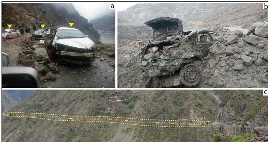
Fig. 2 Impact of rockfalls and debris flows on traffic and travellers: a Rockfall near Dassu crashes cars. Yellow arrows indicate crashed cars (KKH Updates 2016). b Debris flow trapped a car along the KKH. c Small debris flow blocked the highway for couple of hours, and two yellow lines show long line of vehicles on one side of deposit
