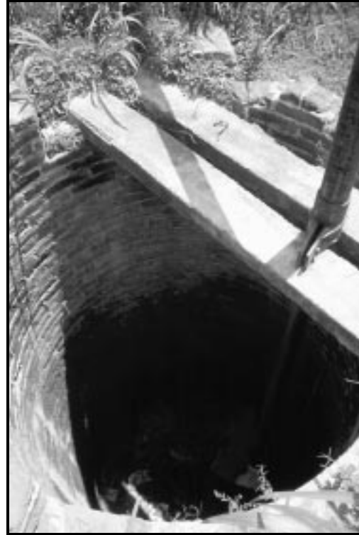
Fig. 95 Former dug wells near El Jabali later on deepened as vertical turbine pump wells
